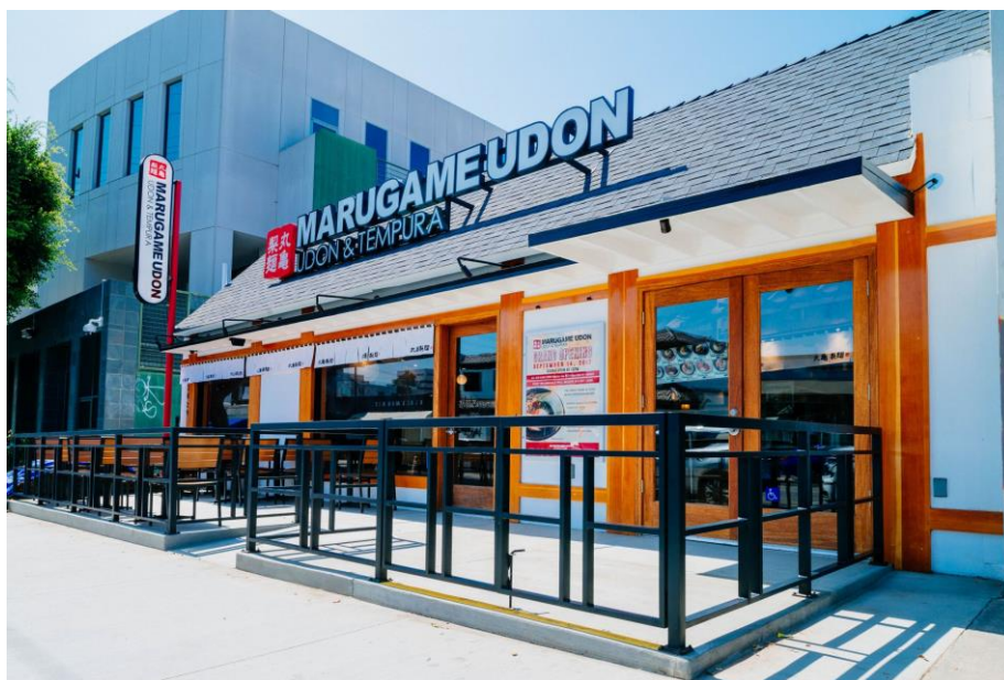
MARUGAME UDON Sawtelle store 外観
